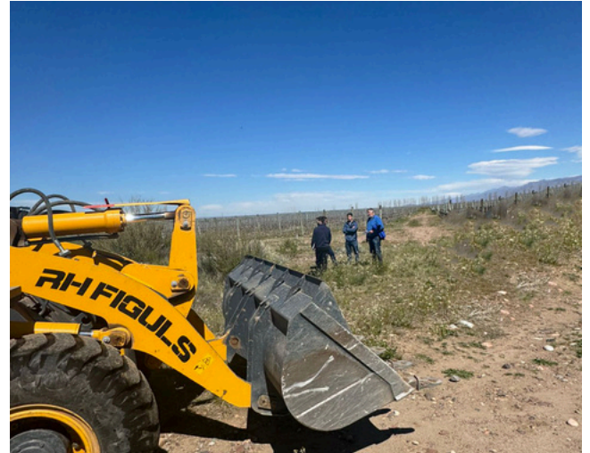
The backhoe beginning the earthmoving work
